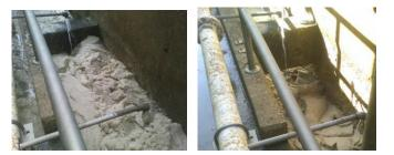
ADDED AS RECEIVED – DO NOT DILUTE WITH WATER. **NOFOAM BIO100** SHOULD BE ADDED TO THE PRIMARY EFFLUENT PRIOR TO AERATION OR INTO THE R.A.S. LINE. IF FOAM BLANKET IS GREATER THAN TWELVE INCHES, THE ADDITION RATE OF **NOFOAM BIO100** REQUIRED FOR EFFECTIVE CONTROL MAY NEED TO BE INCREASED TO 10 – 30 PPM UNTIL THE FOAM BLANKET IS REDUCED TO 3 TO 4 INCHES, THEN 0.5 TO 5 PPM IS SUFFICIENT FOR FOAM CONTROL.
